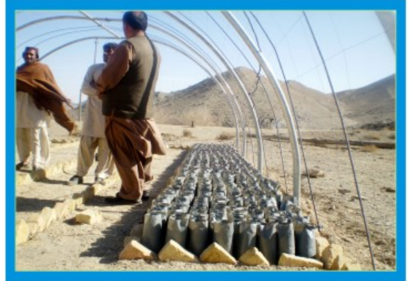
Installation of Green House
