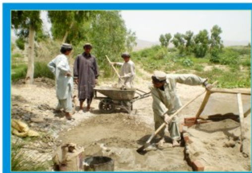
Construction work of water supply scheme in progress
