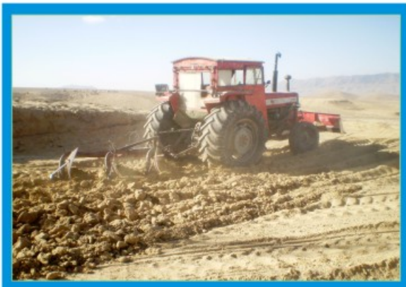
Land leveling for the construction of WHS
