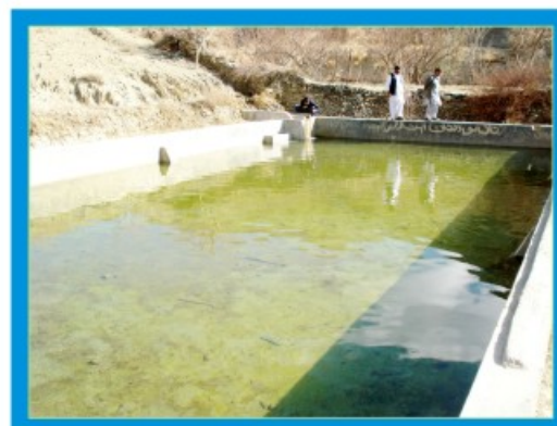
Constructed water storage reservoir in Killa Saifullah
